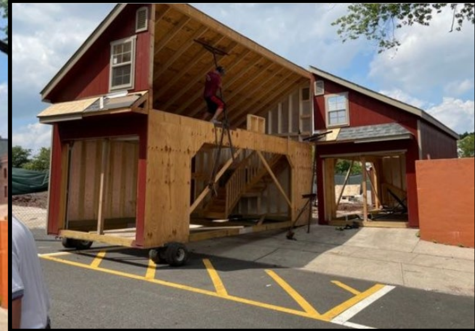
Modular garage installation. Far left – arrival via truck. Center and right – installation in progress.
