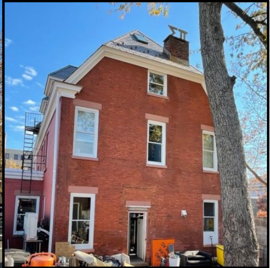
Renovated exterior with new soffits, new windows, restored windowsills.
