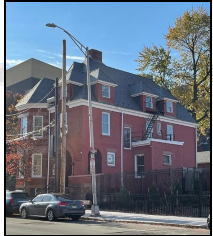
Renovated exterior with new roof, new soffits, new windows, restored windowsills. Left and right also show exterior brick staining.
