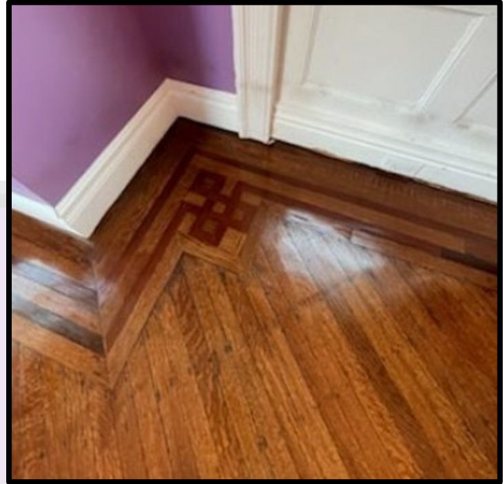
Front Chapter Room refinished flooring
